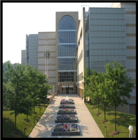
Southern Division Courthouse Greenbelt, Maryland
