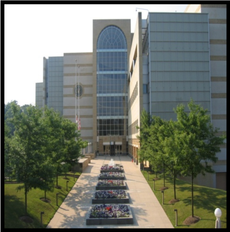
Southern Division Courthouse Greenbelt, Maryland
